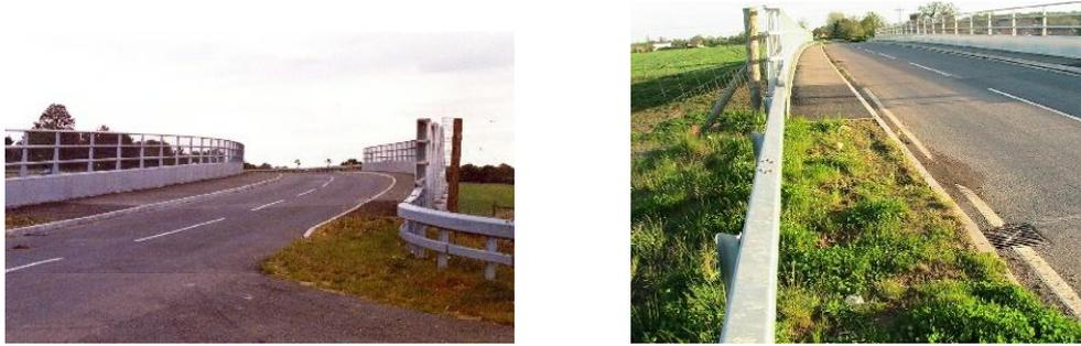
*Photos 1 and 2: Examples of structures accommodating public road traffic leading over A120 Essex, known to be frequented by fallow and muntjac deer. Both structures cross over deer fenced sections of trunk road; base substrate for both is of concrete or tarmac throughout the main span. (Langbein, 2008)*
